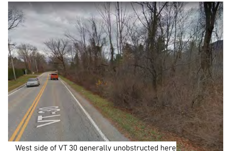
West side of VT 30 generally unobstructed here
