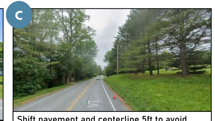
Shift pavement and centerline 5ft to avoid steep slope and trees OR, with property owner support, acquire easement, remove 11 trees, and re-grade slope.
