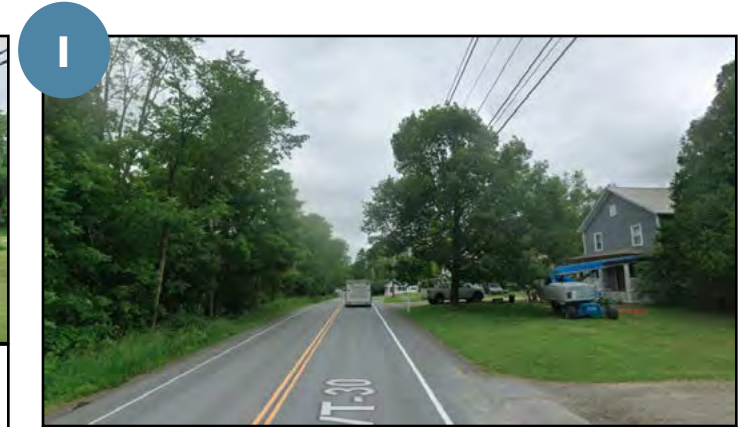
Shift pavement and centerline 7 ft to avoid stone walls and houses on the east side and minimize impacts to the west side.
