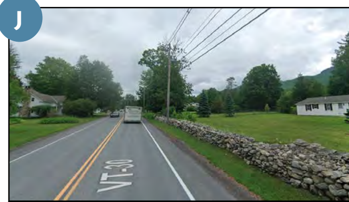
Shift road to avoid ~70 ft of stone wall at 1148 VT 30 (Misai & Misai), currently located within 2 ft of pavement edge.
